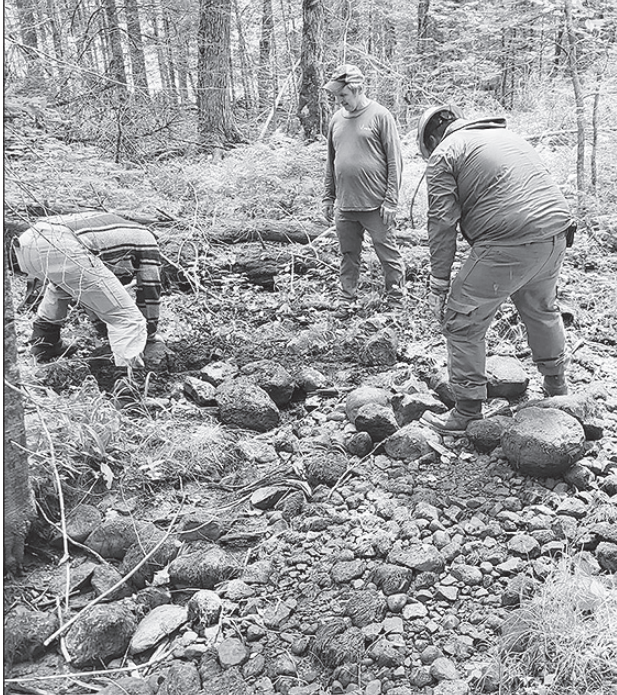
A crew of workers building a stepping stone bridge on a dry creek bed for hikers to cross when the creek is flowing.
