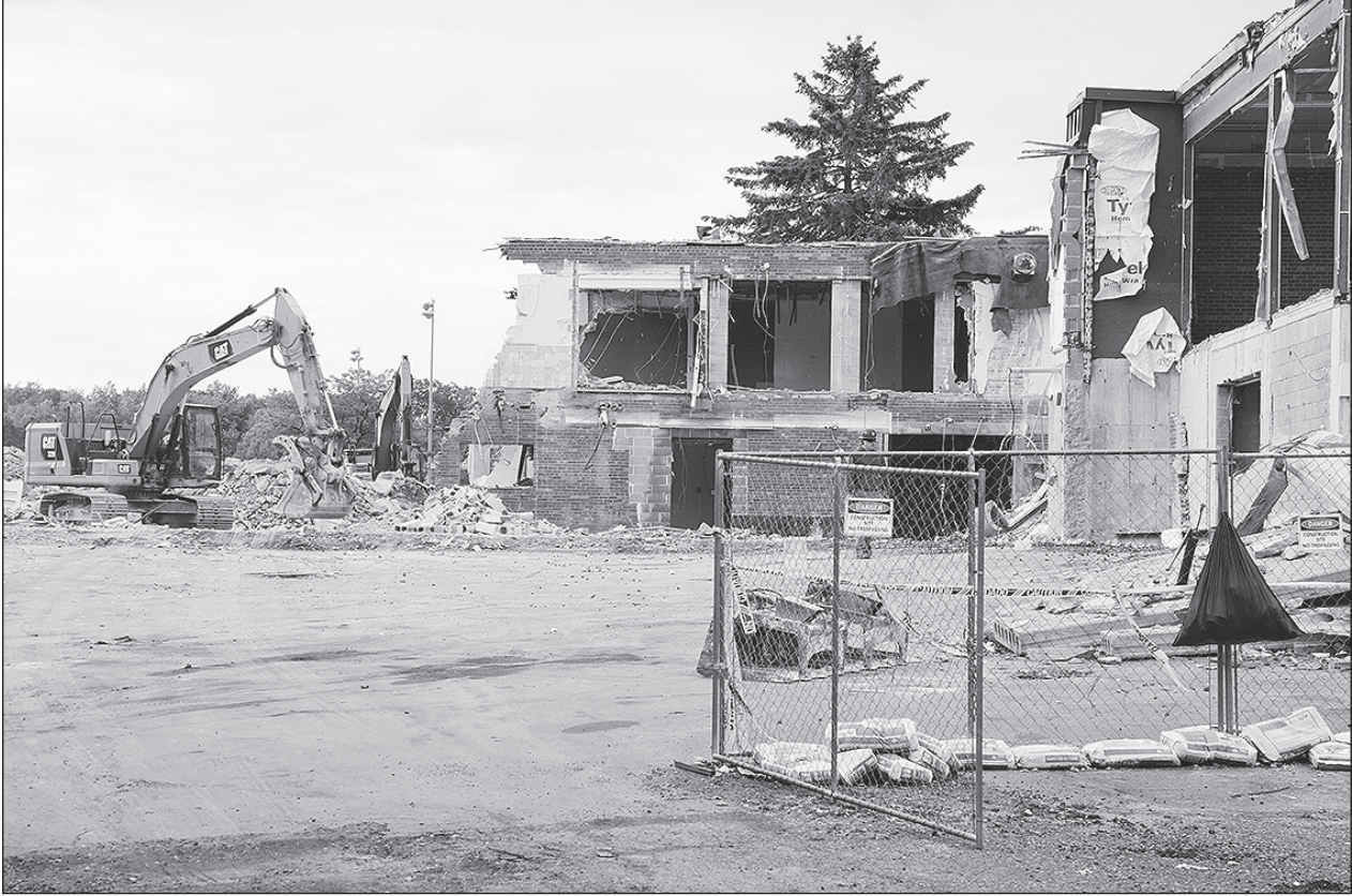
Demolition of the old hospital has been taking place the past couple of weeks.
