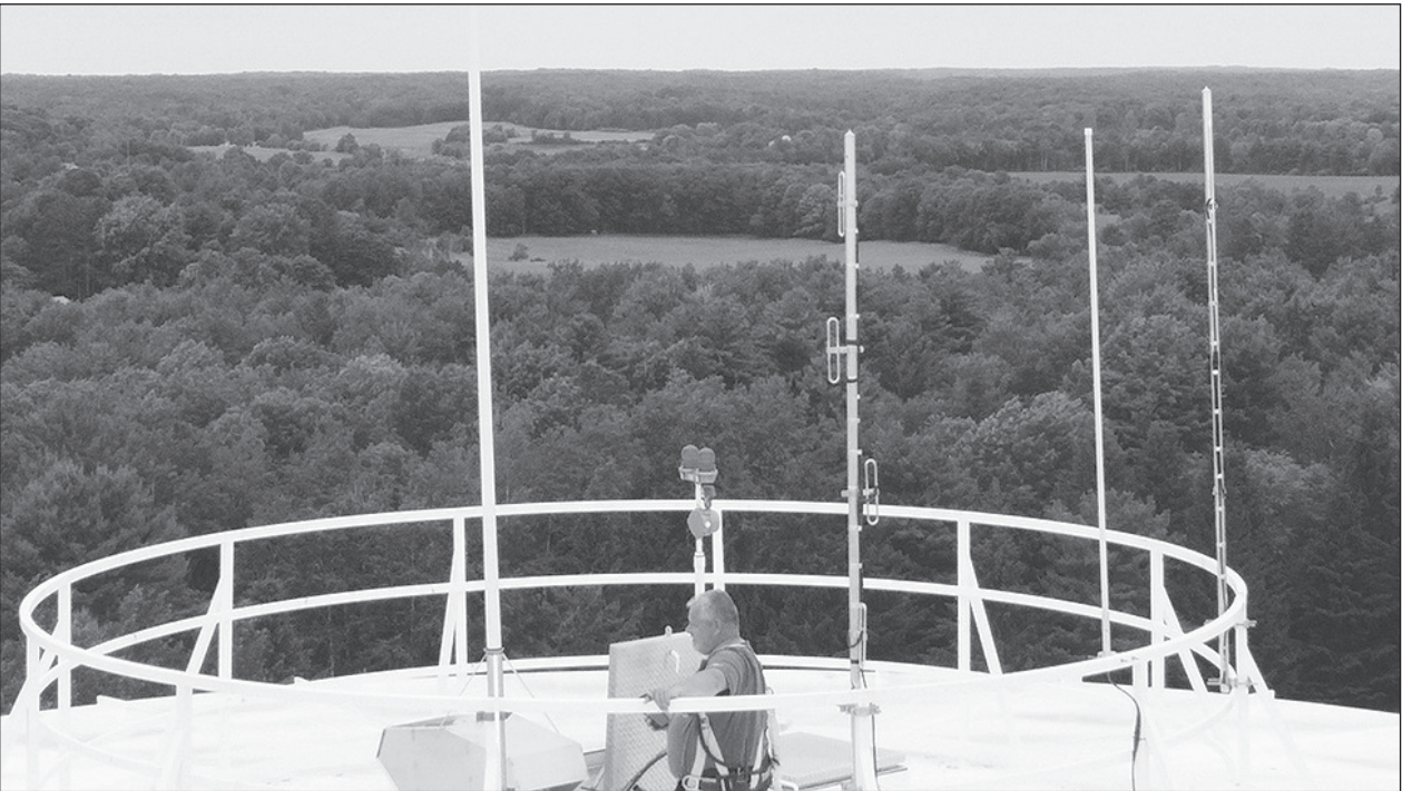
On June 20, Blake Byrd installed a repeater for the Cumberland Fire Department on the Cumberland Water Tower. This will help the department with communication within the department. They will use it for communication when assisting with the Cumberland Rutabaga run/walk, Safe Trick or Treat, and Fire Department training. They will still use Barron County's radio system for calls. Thanks Blake!
