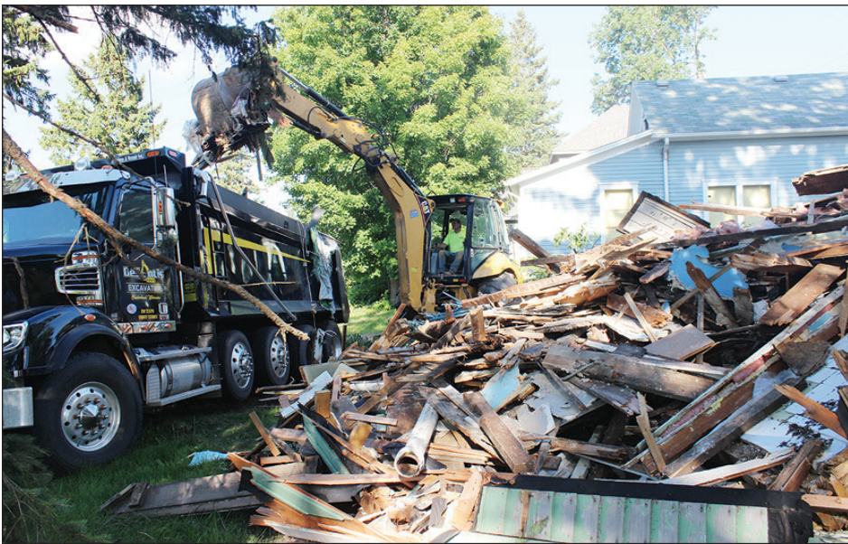
DeSantis Excavating works to tear down and remove three houses starting at 1272 Elm St. to make room for new storm water ponds as well as a possible park area and walking trail.
