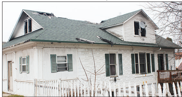
The property to be razed at 1280 2nd Ave
