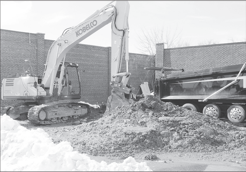
Workers act quickly to repair a water main break between The Verizon Store and Subway on 2nd Avenue on Tuesday, March 2nd.
