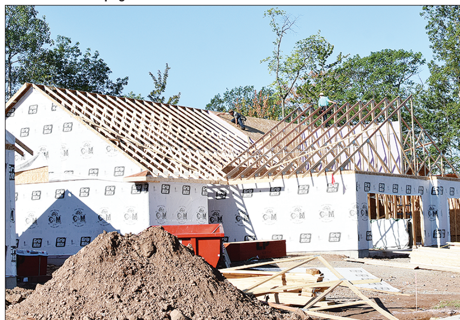
Twin homes are going up in the new development on the city's West side.
