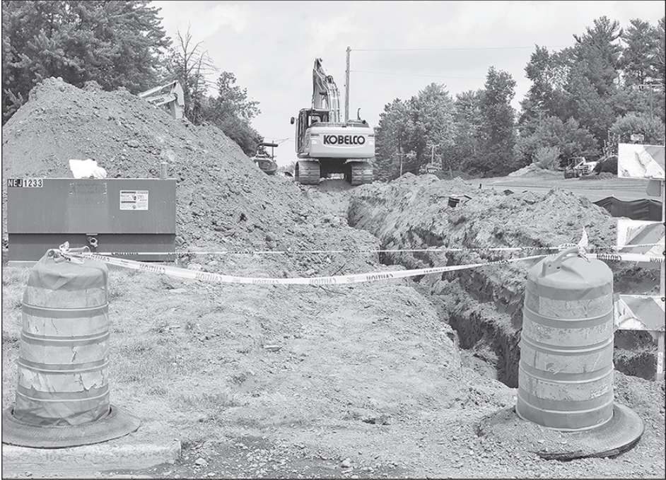
Work continues just north of Jeffery Blvd along Hwy 63 to replace old water and sewer lines. Traffic impact should be kept to a minimum.
