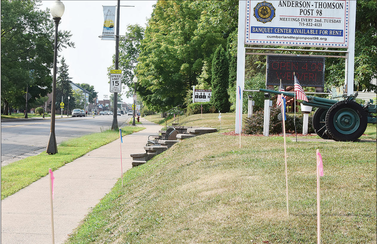
What are all the stakes marking? The DOT placed stakes all along Hwy 63 in town to mark the right of way so it can be surveyed for the 2025 road reconstruction project.
