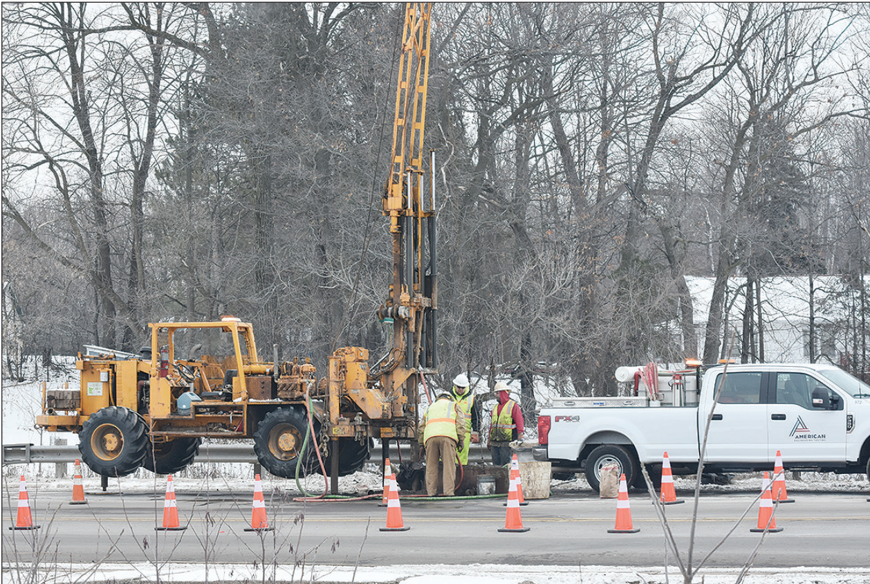
Workers were busy Monday at the Hwy 63 bridge taking core samples for the DOT for the upcoming bridge project scheduled for the summer of 2026.
