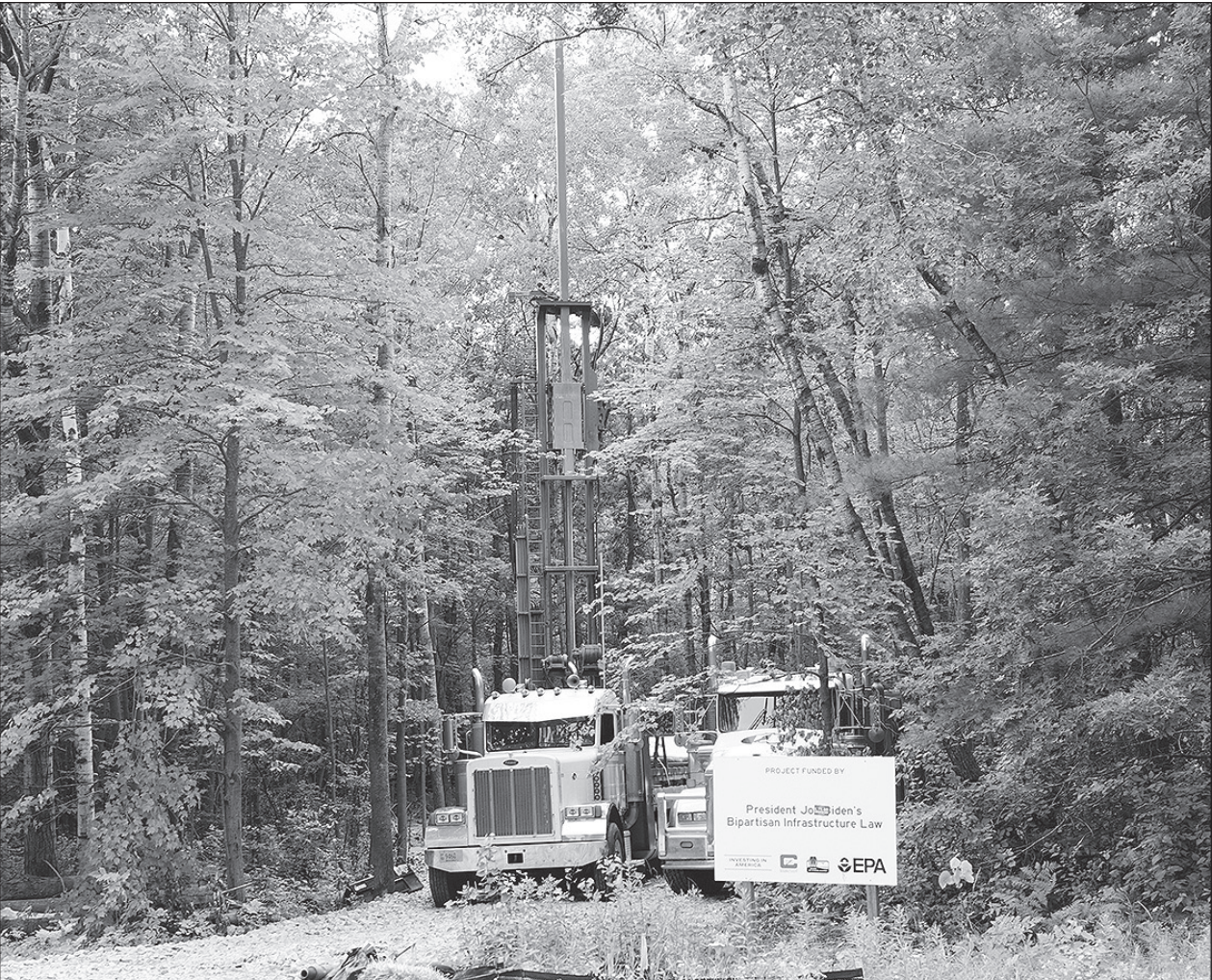
A new city well named #6 is currently being dug on the west side of Highway 48 just north of the city. When operational, the well will produce between 700 and 750 gallons of water a minute. The new well looks to be up and running in the Fall of 2025.
