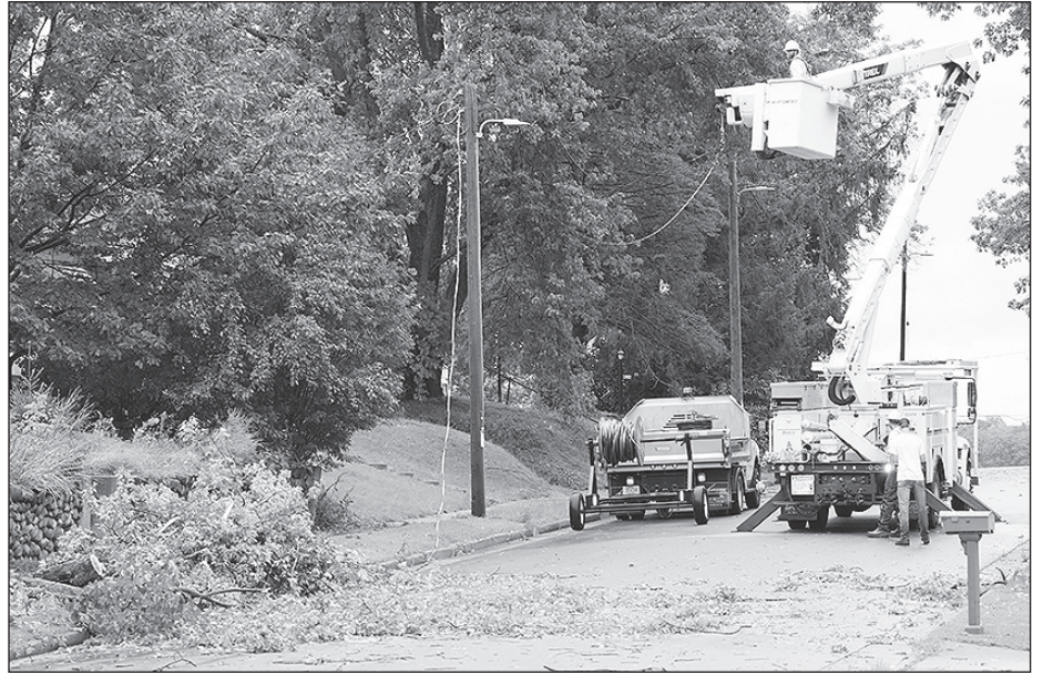
Cumberland Municipal Utility Crews worked on a down power line Tuesday morning on 5th Avenue in Cumberland. Overnight heavy winds brought widespread power outages, and downed trees to the area.
