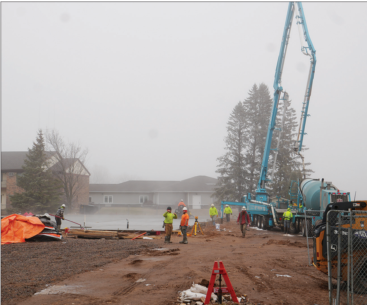
Workers from Northwest Builders pour concrete at the soon to be maintenance building Monday morning as the start of the $32.5 million dollar school referendum project begins. The new maintenance building will act as a temporary learning center for the current west wing of the current high school as the building project progresses.
