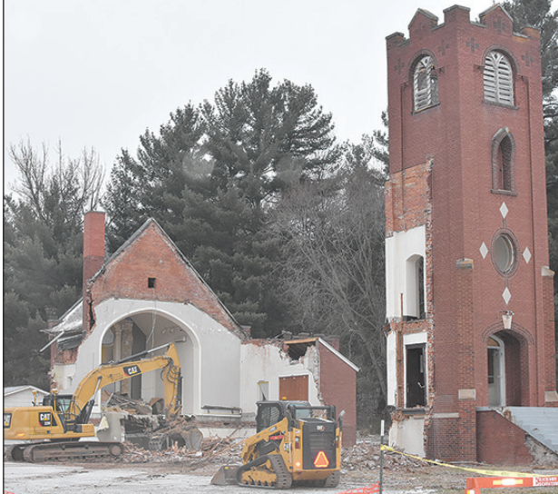
The demolishing of St. Anthony Catholic Church.
