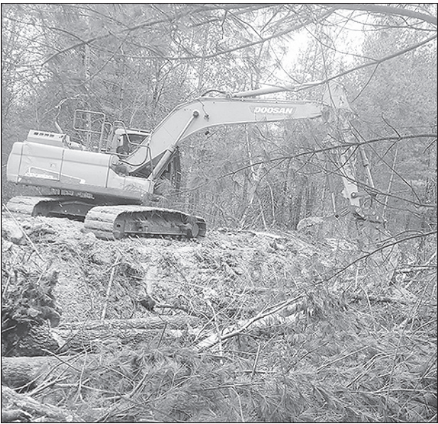
Excavators are used to remove the trees and place them in the ditches.
