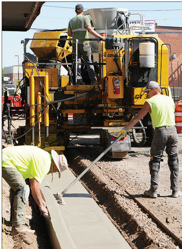
Road construction workers smooth out a new section of curb Tuesday morning as they continue to steadily make their way north.
