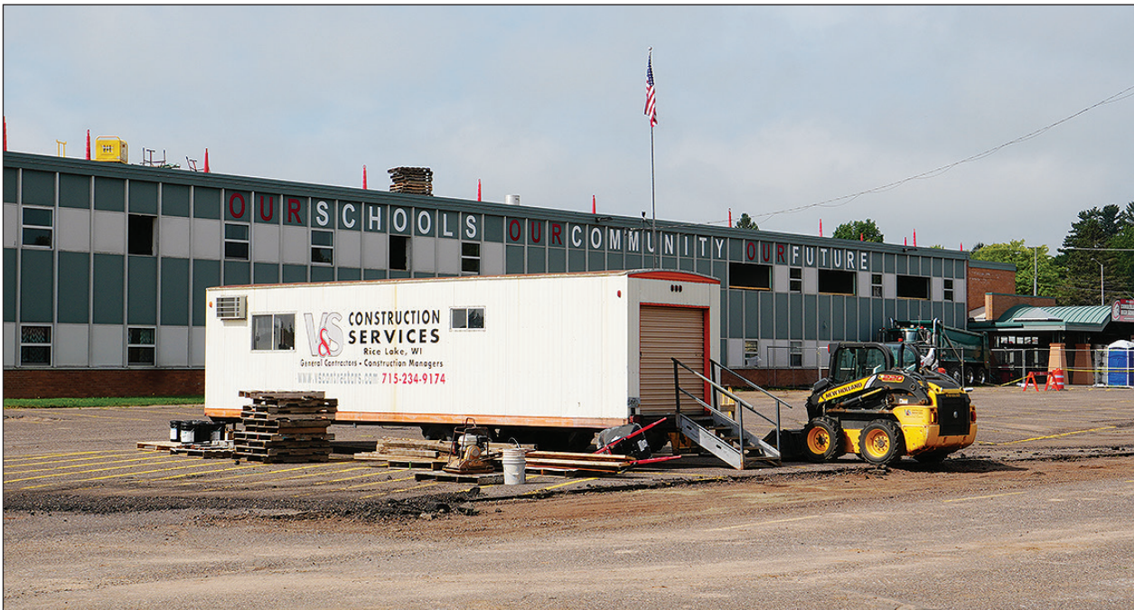
Construction is in full swing at the Cumberland High School. The 32 million dollar project will take up to 15 months for completion.
