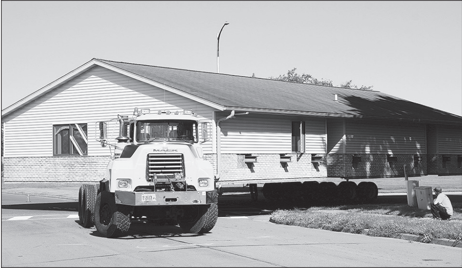
The old Cumberland School District Office building was sold to a private owner and moved on Monday, June 30th to a location on Berdan Street. It was quite the operation watching workers maneuver the building around the corner of 8th and Berdan Street.
