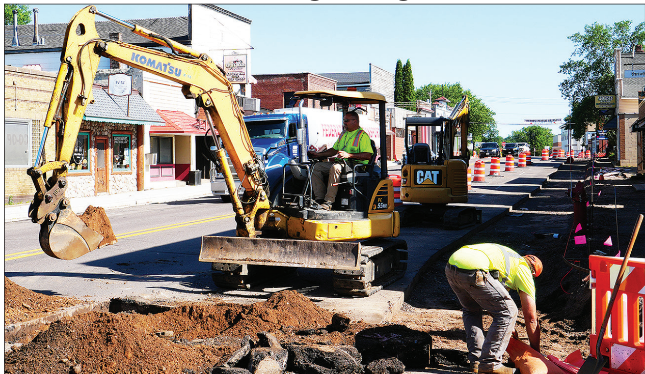
Work continues to progress on the Hwy 63 road construction project.
