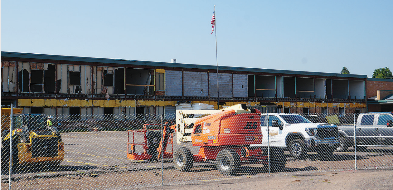
If you didn't know CHS was undergoing a major renovation and just saw this photo you might not know what building you were looking at. As the old saying goes this sometimes must get worse before they get better.
