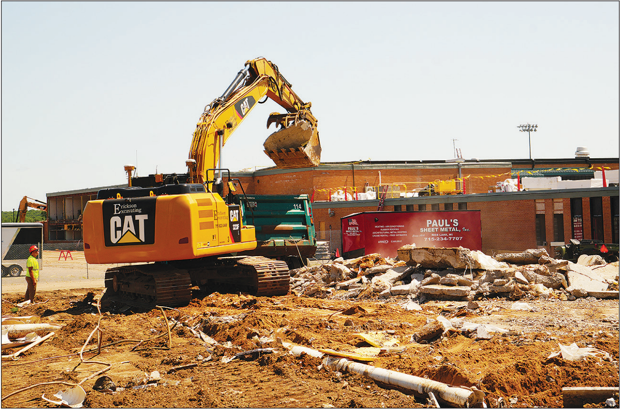
Work continues at Cumberland High School.
