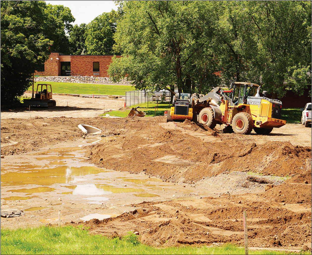
Progress is being made on Marshall Street and First Avenue behind Cumberland Elementary.
