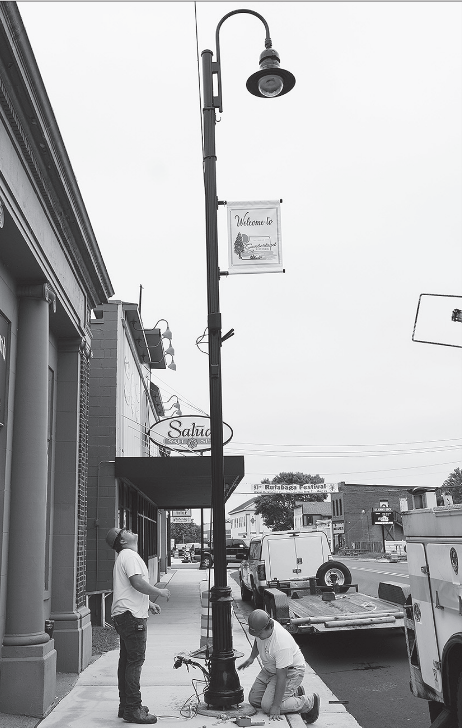
The new street lights are being installed up and down Main Street and should be good to go for Rutabaga Festival and beyond. The new lights look fantastic!
