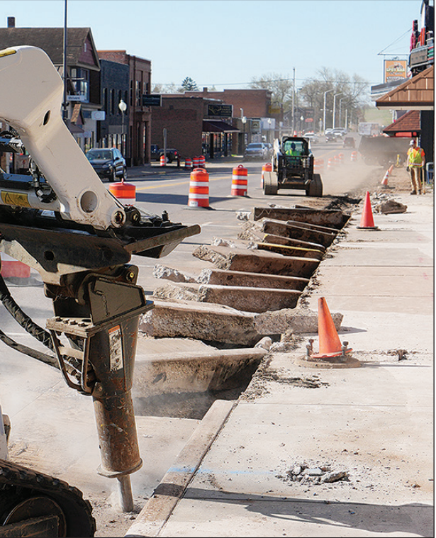
Road Construction gets underway.
