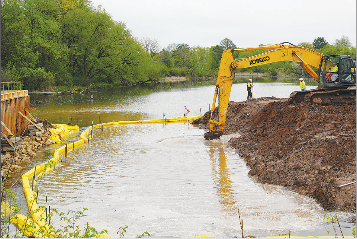
THE US HWY 63 BRIDGE REPLACEMENT PROJECT IS MOVING ALONG. EVERY WEEK WITH GOOD WEATHER HELPS TO SHORTEN THE LENGTH OF THE PROJECT WHICH IS EXPECTED TO BE COMPLETED IN EARLY SEPTEMBER.
