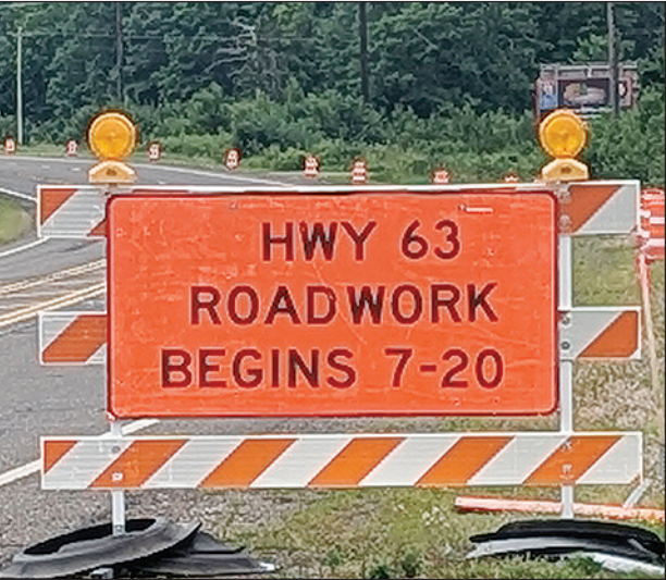
THE US HWY 63 ROAD CONSTRUCTION PROJECT FROM CUMBERLAND TO TURTLE LAKE BEGAN ON MONDAY, JULY 20TH AND IS EXPECTED TO LAST UNTIL NOVEMBER. HWY 63 WILL REMAIN OPEN TO TRAFFIC THROUGHOUT THE CONSTRUCTION PROCESS WITH FLAGGERS DIRECTING TRAFFIC.
