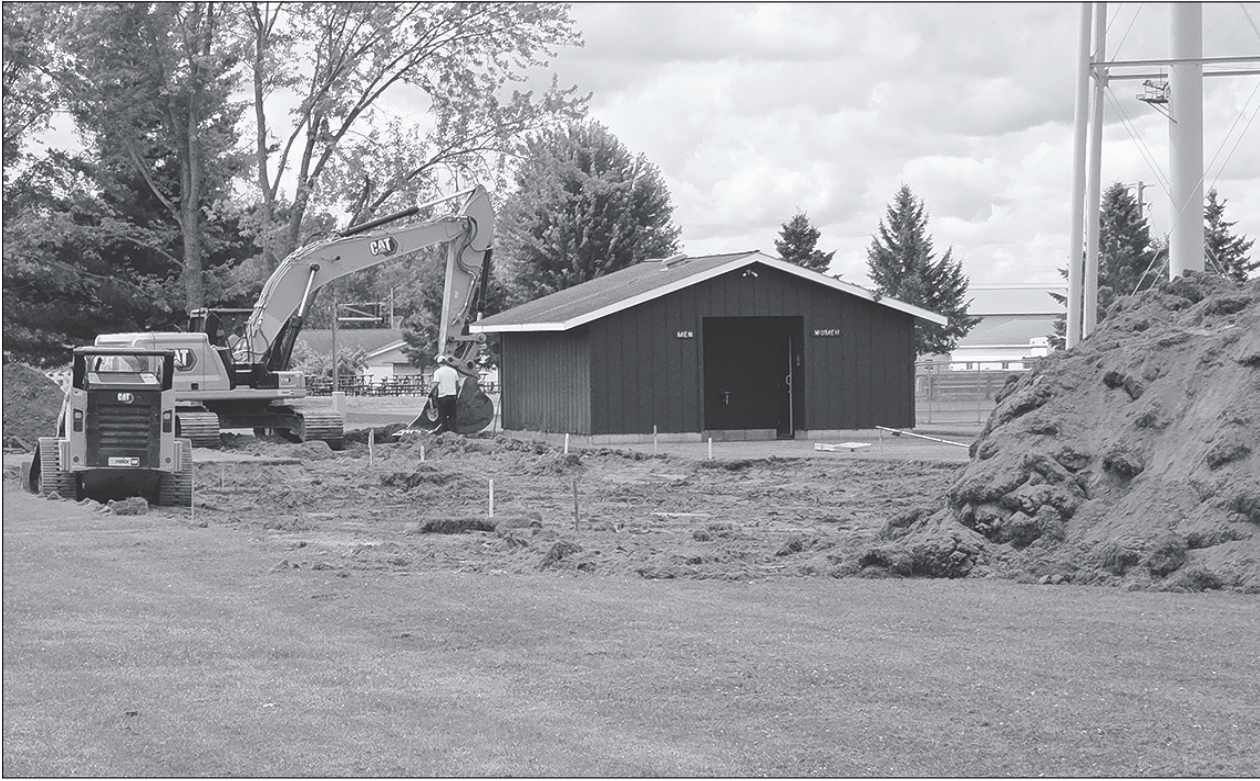
Construction began on Wednesday, July 22, 2026 on the FEMA-funded project to build a community safe room storm shelter at Shadyside Park in Almena.
