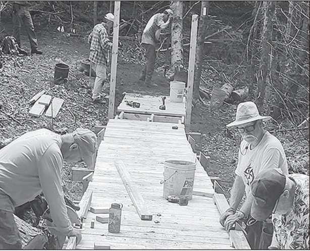
Building this 52-foot section of boardwalk was a physical and challenging task by Ice Age Trail volunteers.
